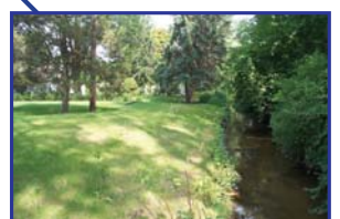
The City of Novi received Rouge Project funding to conduct a streambank stabilization project using bioengineering upstream of the Northville Mill Pond.
