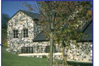
Linden Park in Birmingham is the site of one of three combined sewer overflow control basins in Oakland County.
