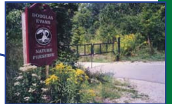
The Acacia Park combined sewer overflow control basin is located at the Douglas Evans Nature Preserve in Beverly Hills.
