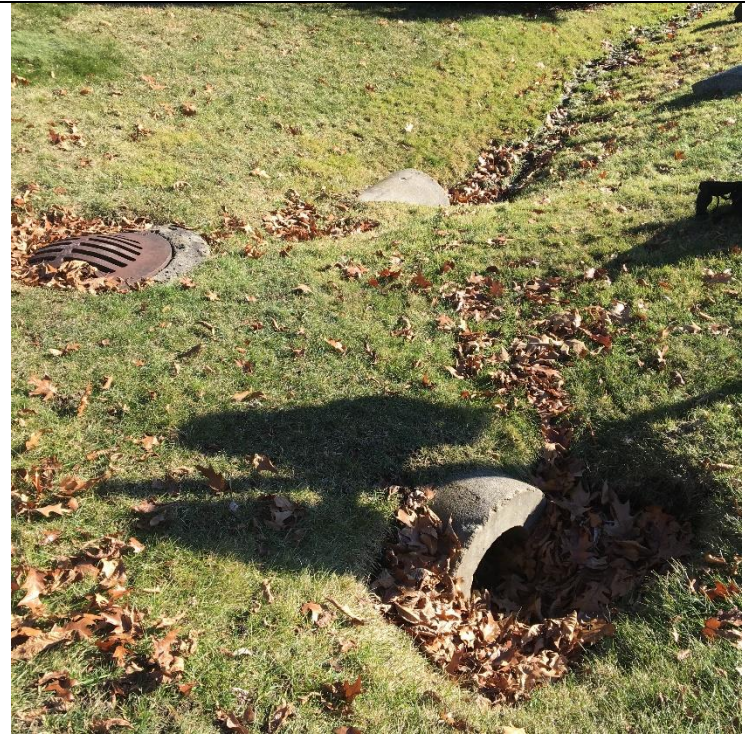
Beehive CB on Steeplechase. Connects Rd drain ditches. Flow in E. ditch line. Sampled
