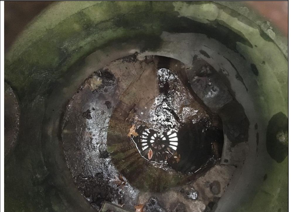
CB connects inlets for Whippers LN. & Hunt Master to MH 7316. Ponding at E outlet
