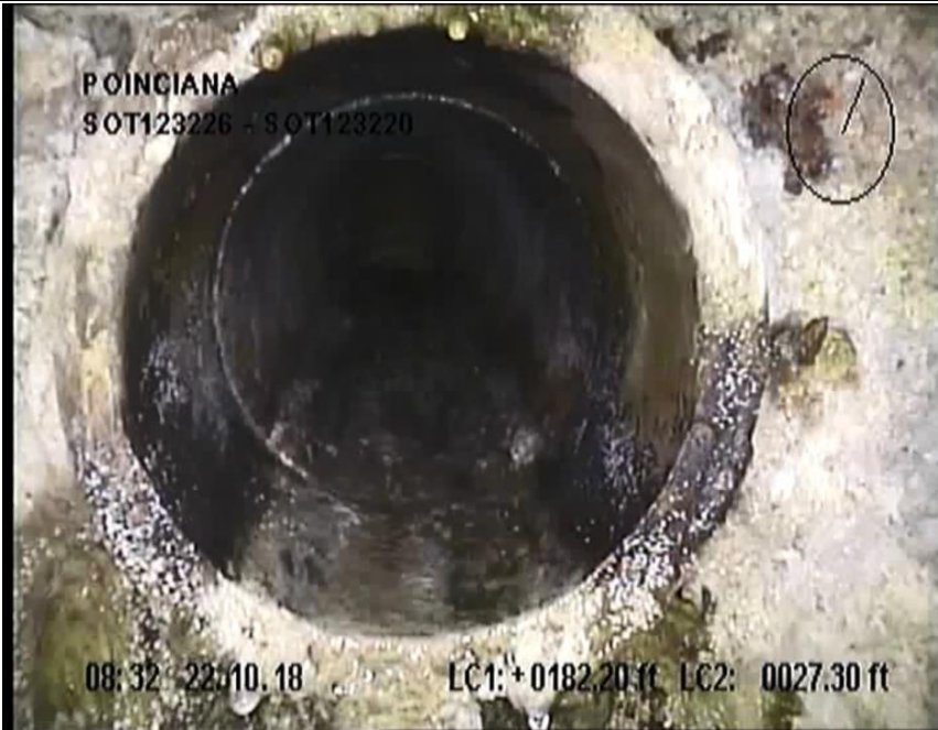
6" Clay Tile Tap 182.20 ft. S. of MH SOT123226 @ 21365 Poinciana
