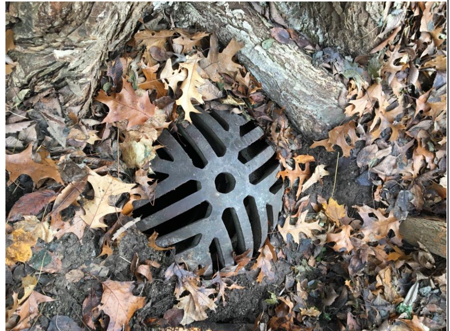
Dover 3 CB located E. of drive at 4725 Dover in woods. Beehive is locked in by tree roots
