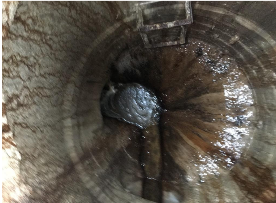
MH 408 . Flow from N. is pooled at elbow going E. Brown with suds, staining on MH wall
