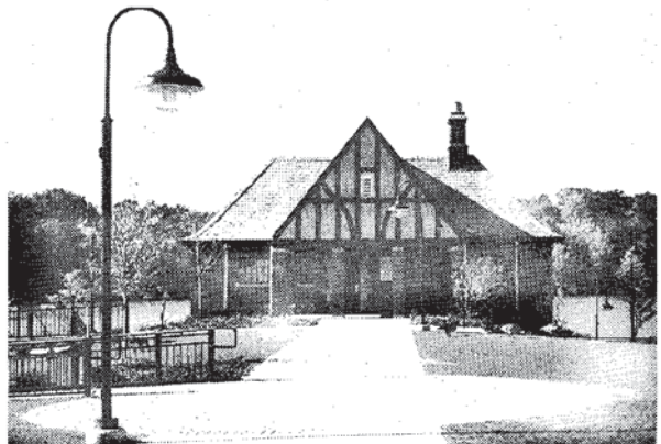
Comfort station, Middle Rouge Parkway Improvement Project
