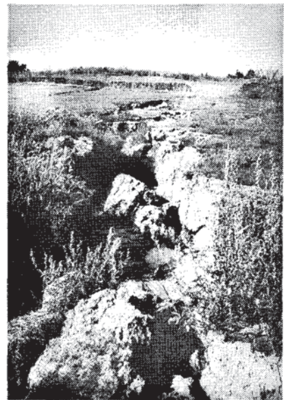
Erosion at a construction site
