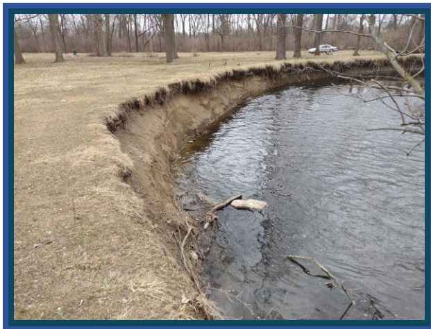
Figure 4. Sample observation from Inkster general site assessment. At Inkster Park, a bare riverbank with severe erosion was observed.
