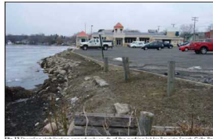
Site 13 Shoreline stabilization opportunity south of the parking lot for Bayside Sports Grille Restaurant
