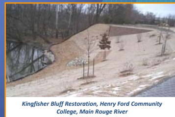
Kingfisher Bluff Streambank Erosion, Henry Ford Community College, Main Rouge River
