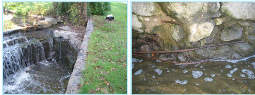
Existing Conditions: Failing Dam
