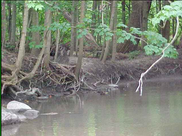
Stream Bank Erosion
