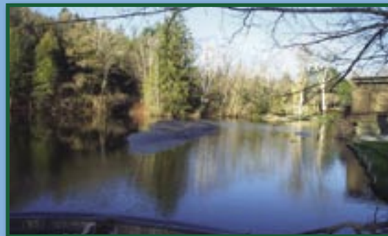
Danvers Pond Dam
