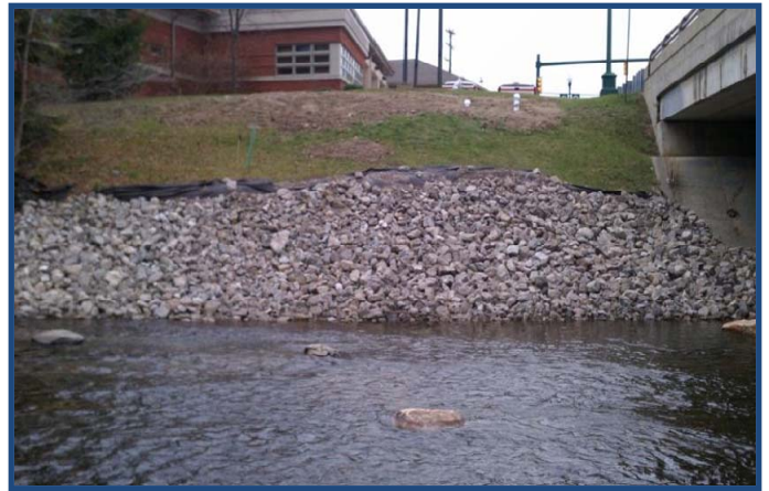
Bank stabilization after restoration
