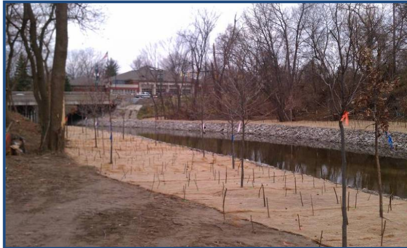
November 26, 2012: View from downstream end of constructed south bench looking northwest with erosion control blanket and live stakes installed
