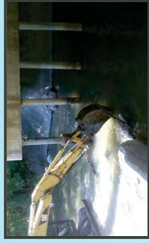
Removal of the dam sill.
