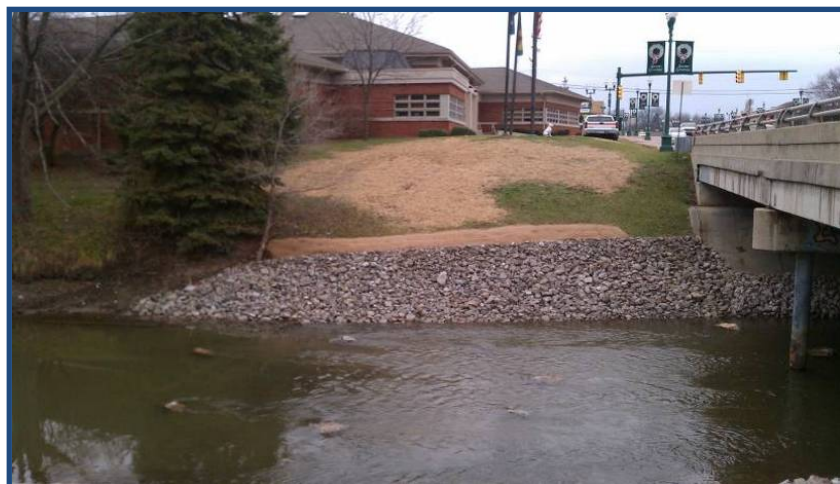
December 17, 2012: North bank upstream (west) of bridge, note rock stabilization, erosion control blanket, straw mulch
