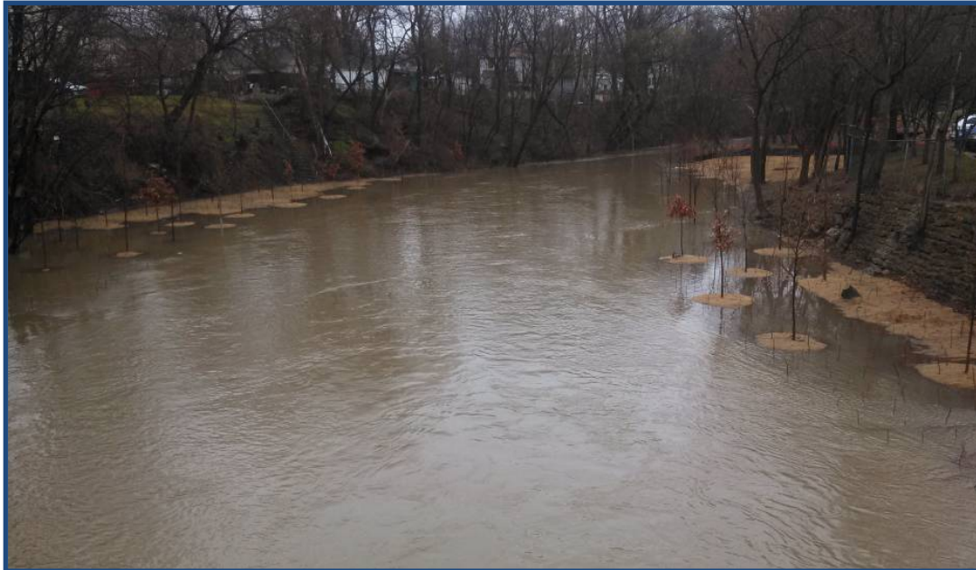
April 11, 2013: View from bridge looking downstream (east) after sequence of rain events, note, bankfull benches overtopped
