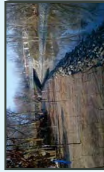
With tree planting complete, seed was placed and erosion control blanket was installed on the bankfull benches. Then, live stakes were installed.
