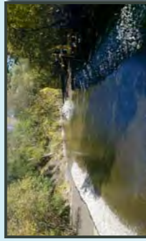
Sand bankfill was placed behind the stone toe. Geotextile fabric was used between the stone toe and the sand bankfill.
