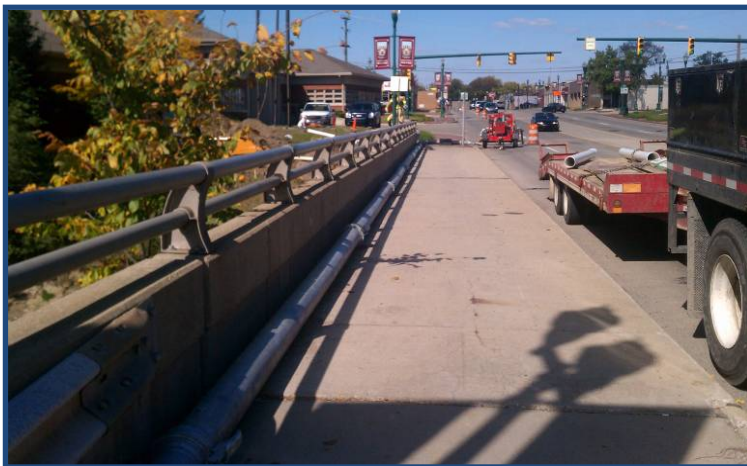
Diversion pipe used during sewer connection work
