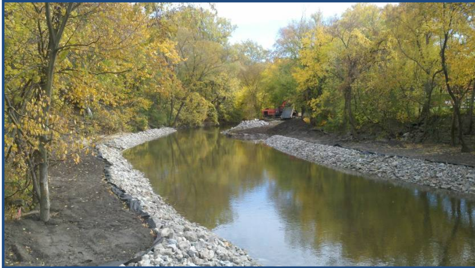
October 24, 2012: View from bridge looking downstream (east). Note: rock at north bench complete
