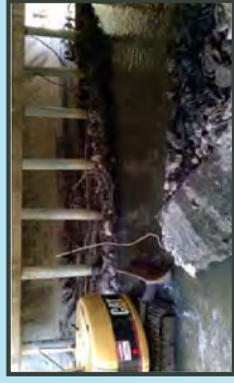
Lowering of water level at the dam by notching the dam.
