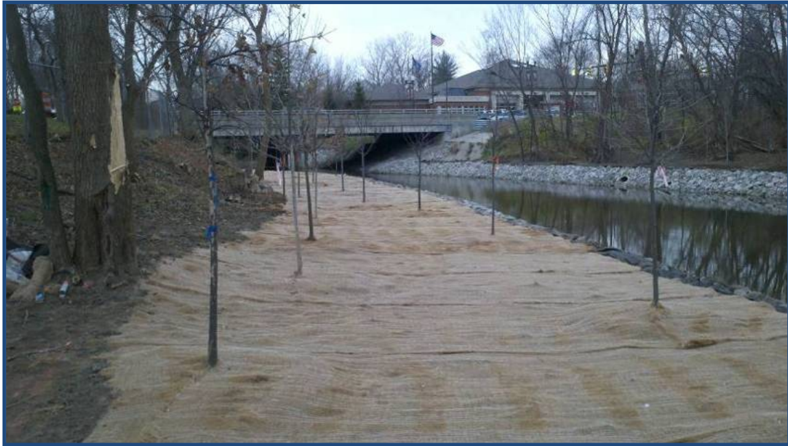
November 19, 2012: View from downstream end of constructed south bench looking upstream (west) and erosion control blanket installation
