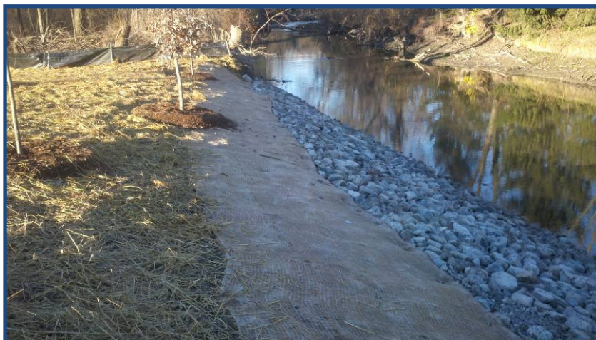
December 5, 2012: South bank upstream (west) of the bridge. Note: rock toe, graded top of bank, erosion control blanket, trees, straw mulch
