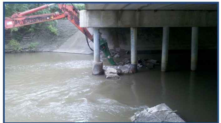
Spillway removal
