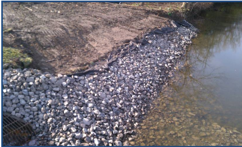
November 14, 2012: View from bridge looking upstream at south bank. (southwest). Rock toe and shaping of top of bank
