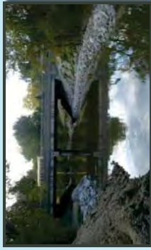
Sand bankfill was placed behind the stone toe. Geotextile fabric was used between the stone toe and the sand bankfill.
