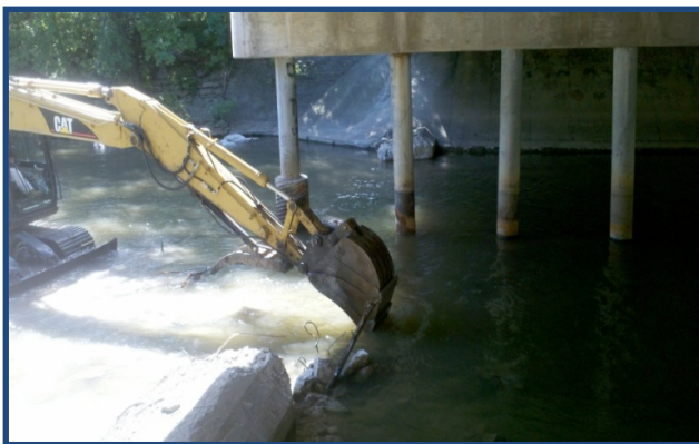
Spillway removal
