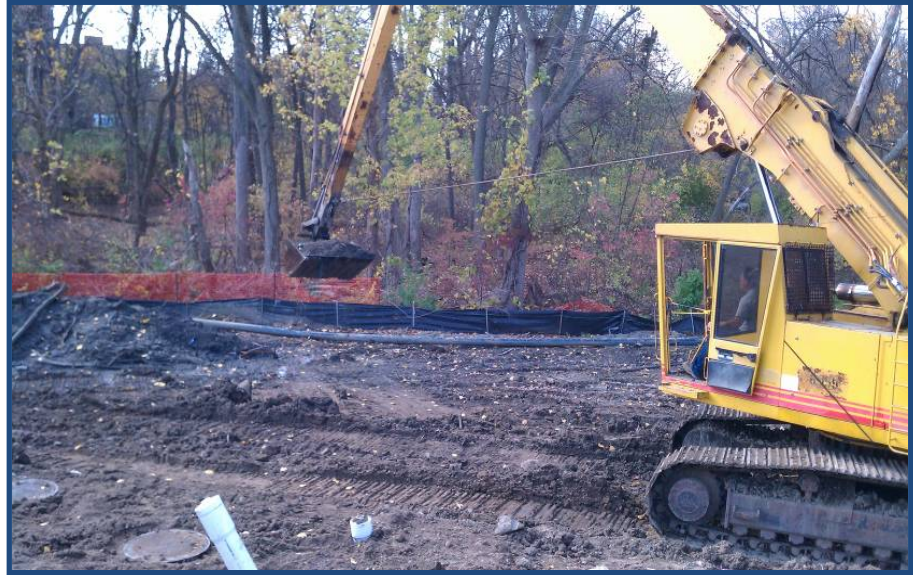
Excavating upstream of the bridge. Note old sanitary sewer pipe in staging area
