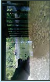
The rock for the riffle was placed under the bridge. A 6" thick layer of smaller stone was placed first and overtopped by larger rock.
