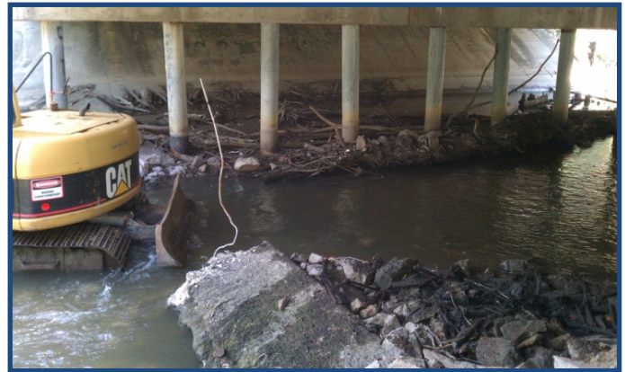
Notching of spillway
