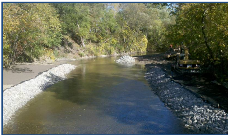
October 11, 2012: View from bridge looking downstream (east). Note: topsoil placed overtop of sand backfill.
