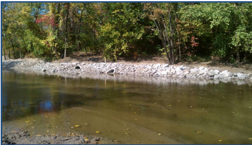
North bankfull bench, downstream of bridge, view looking northwest. Note: two newly installed stormwater outfalls
