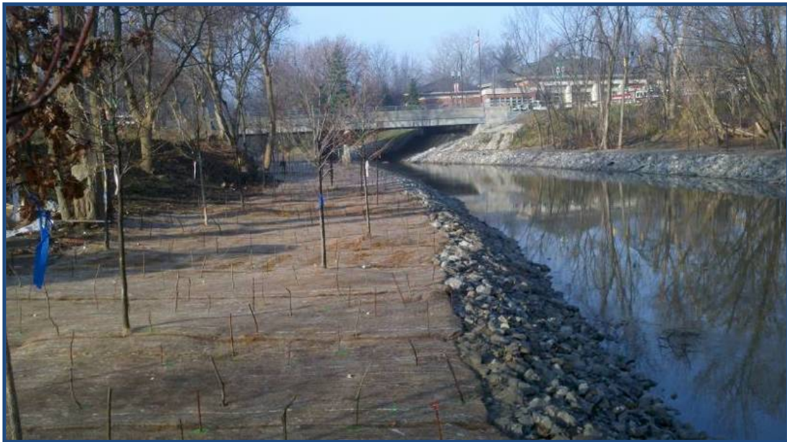
November 21, 2012: View from downstream end of constructed south bench looking upstream (west) and live stakes installation
