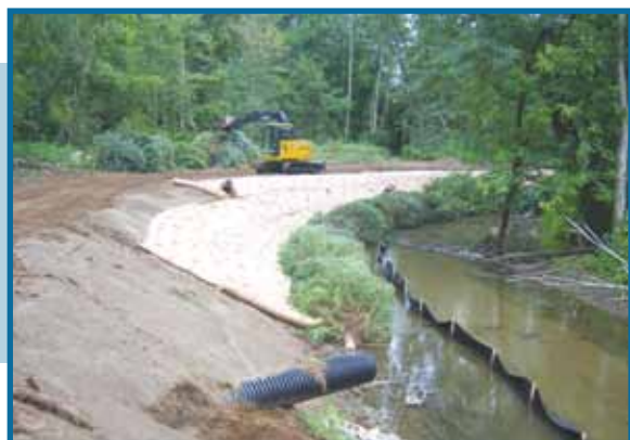
Installation of soft engineering techniques such as erosion control blankets and trees
