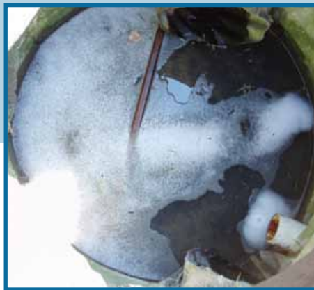
Illicit connection discharging soapy water to a storm sewer
