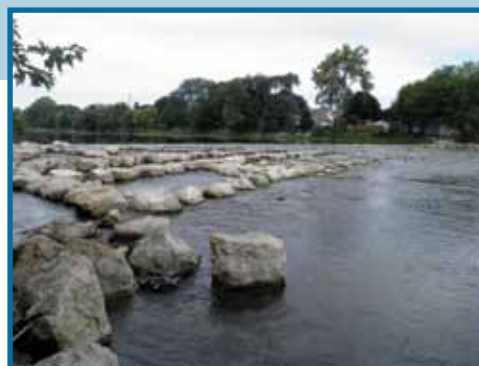
Rock arch rapids installed
