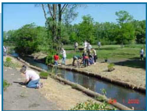
Streambank stabilization in Firefighters Park
