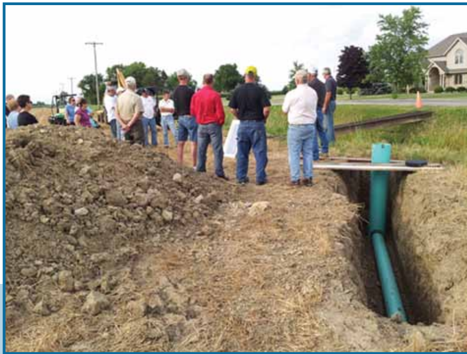
Drainage water management structure with Garage of Knowledge participants
